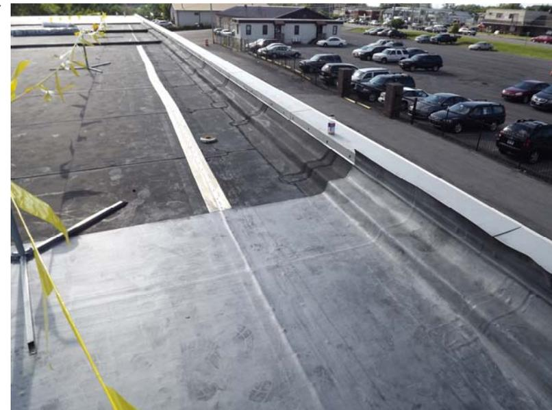
New 2001 Co. wind vented 60 mil C-EPDM installed directly over an existing totally adhered EPDM.
