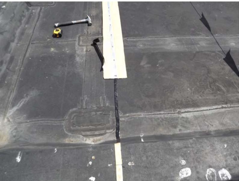
7. Unroll the largest EPDM sheet that can be handled over the existing roof. A 30x150 folded once with a 15' crease covers large area.
