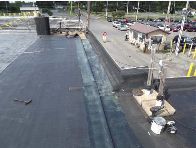
14. Totally adhere the remainder of the field membrane to the existing roof and its angle change terminations with rubber to rubber adhesive.
