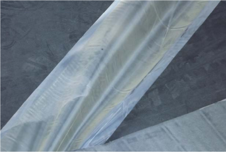
A close up of the angle that the paper backing is supposed to be pulled at.
