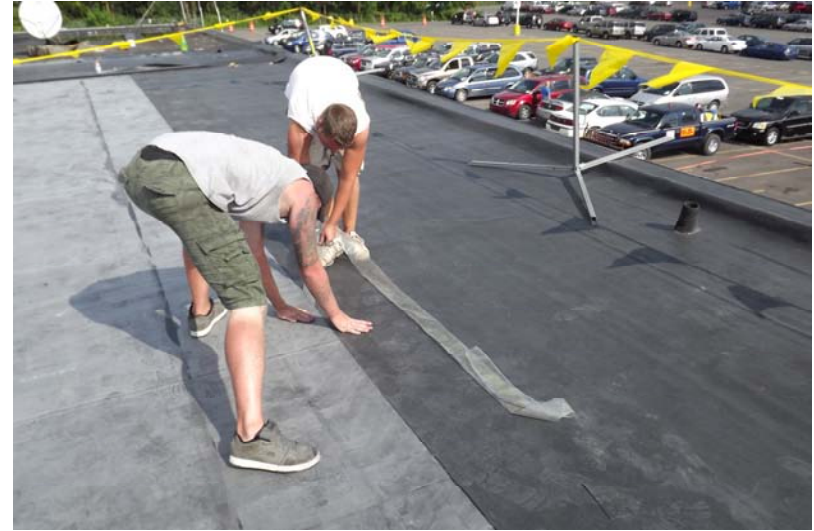
As one man pulls the paper backing, the other one presses down on the top membrane affixing it to the bottom sheet.
