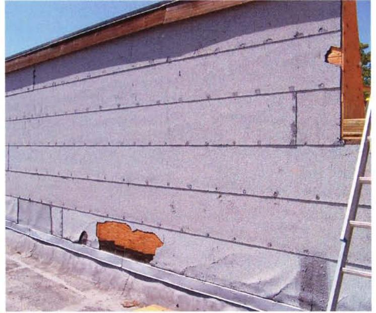
On parapet and interior facing mansard flashing walls that need to release condensation and breath out water vapor, the patented 2001 Company **Wind Vented Vertical Wall Flashing System** controls flashing membrane backside condensation and moisture build-up.
