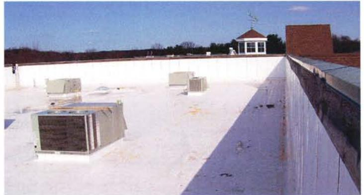
This patented wind vented wall flashing technique weeps condensation out of a vertical wall like traditional brick wall waterproofing and ventilates mansard peak hot air and water vapor build-up in wind uplift vortex intensity areas on vertical walls.
