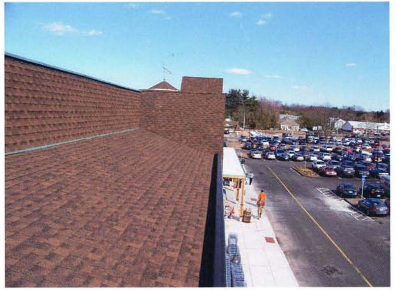
Water vapor build-up in the decorative mansard cavity wall will condensate on the back side of the wall flashing and constantly wet the wood and rust the nail. The sun-facing mansard front heats up during the day causing hot humid air to move to the cold north face interior wall and condensate causing erratic dripping on the store's inside drop ceiling but never when it rained. The wall flashings were constant maintenance and the plywood wall would buckle and rot. See above pictures.
