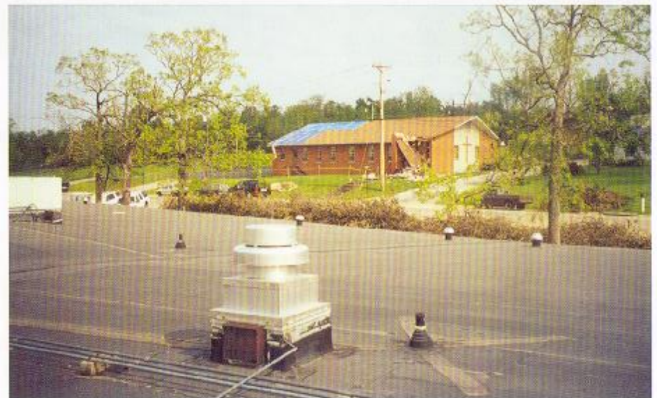
Church across the street had a wall collapse, along with roof edge and peak blow off.
